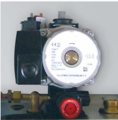
Pump body with built-in air vent
